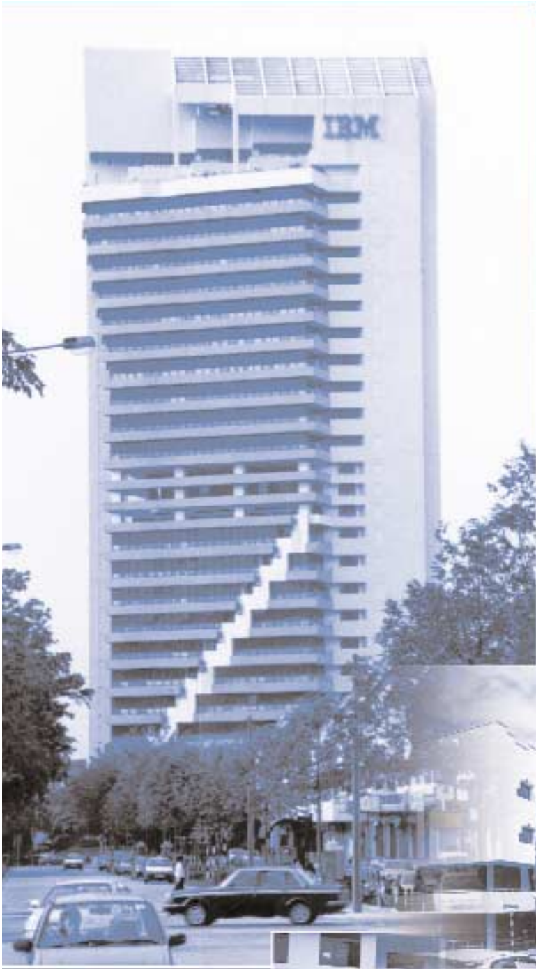
24-Storey Office Building known as Plaza IBM Taman Tun Dr. Ismail Kuala Lumpur
